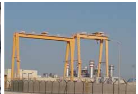
Gantry Crane (Oman Barka II Project)
